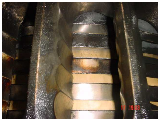
Minor blow-by past 1 st ring of Unit 4
